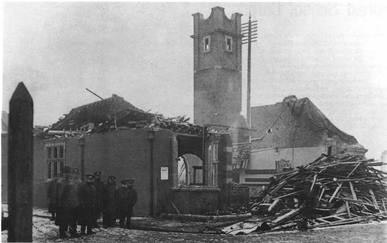
The Silvertown Fire Station pictured after the explosion at the nearby Brunner, Mond and Co. munitions factory on
