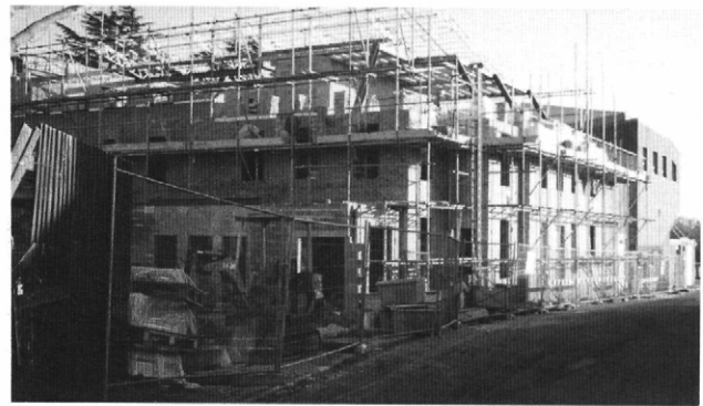
Work-in-progress on the Jenkin Wing.
