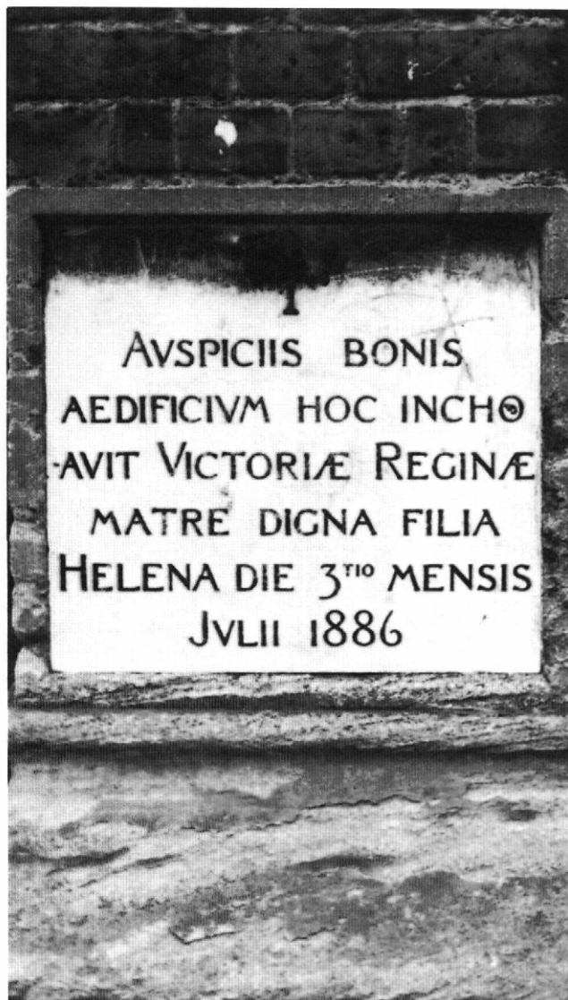
Foundation Stone of the Dining Hall, reminding us of the July day of 1886 when Princess Helena visited the School.
