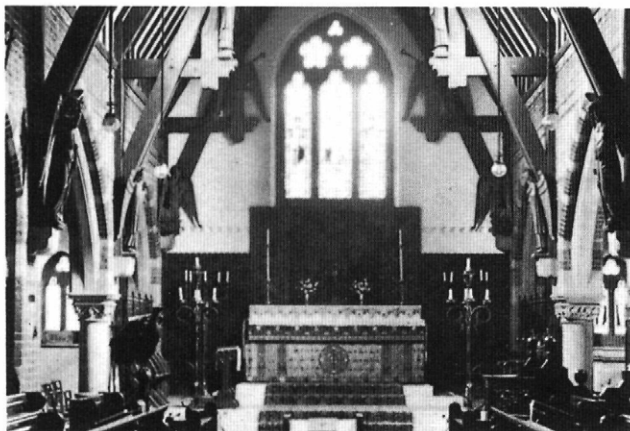
The Chapel. Built at the end of Gilderdale's headmastership, though much enlarged later on. This photograph was taken during the nineteenth century but after the building was enlarged at the east end in 1875. The twentieth century photograph shows the main changes: namely electric
