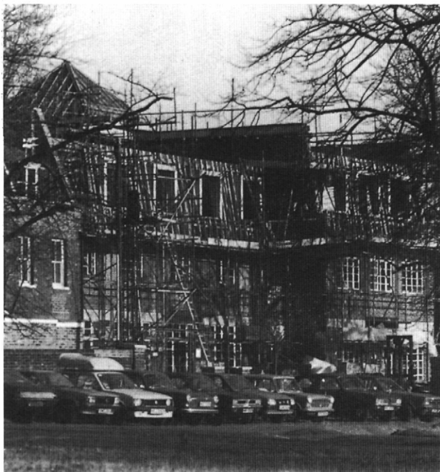
The 1980s saw the expansion of Junior School — much needed classrooms were provided as a third storey was added to the existing building during Winter 1983-1984.
